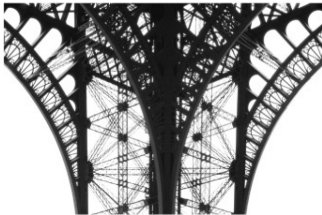
13. Structural hierarchy, common in nature's materials, is exemplified in the Eiffel Tower.
